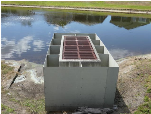
Stormwater Drainage Control Structure
