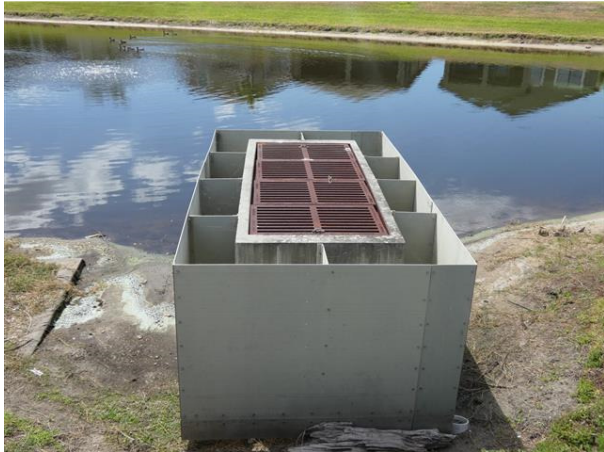
Stormwater Drainage Control Structure
