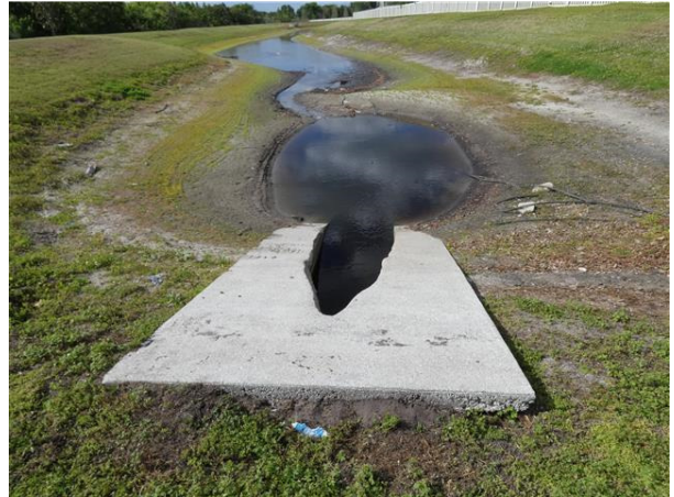
Stormwater Drainage Mitered End Section
